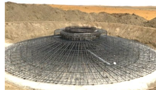
風力発電所(Blue Hills Wind Energy Project)
